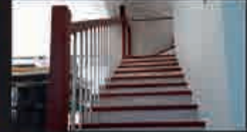
Wooden stairs & stone cladding
