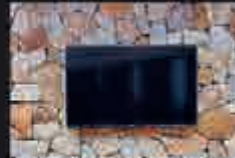
Natural loose stone cladding
