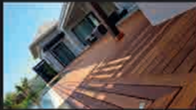
Pool Solid wood decking
