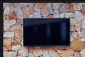
Natural loose stone cladding
