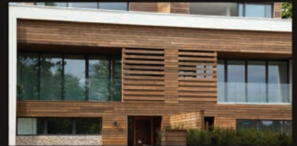
Facade timber cladding
