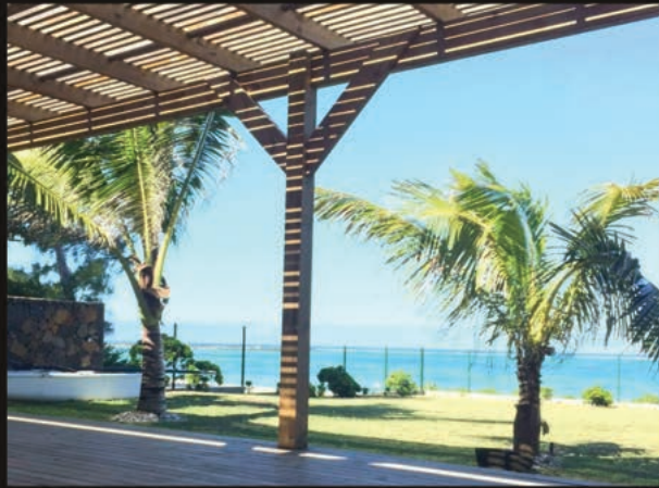
Timber pergola & Decking
