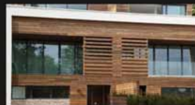
Facade timber cladding
