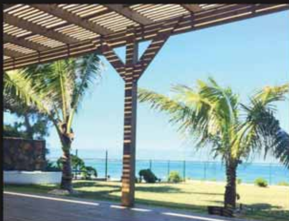
Timber pergola & Decking
