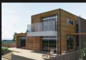
House exterior timber cladding
